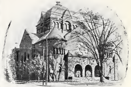
The Temple, built 1892, corner Scovill avenue and E. 55th street
